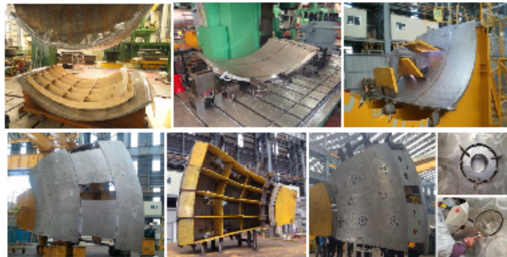
Progress of Upper Segment for the First Sector
